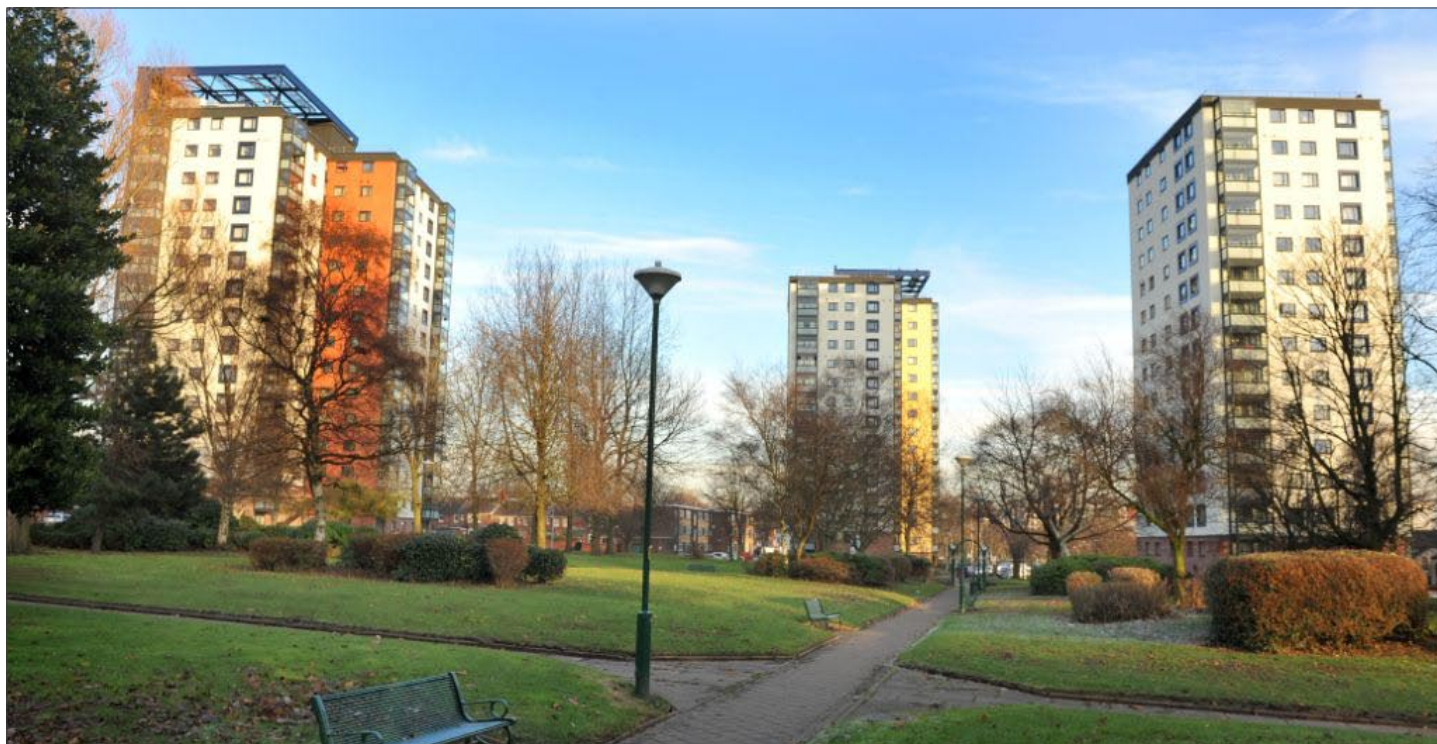
Kemball, Craunton and Cremer high rise blocks after refurbishment.
